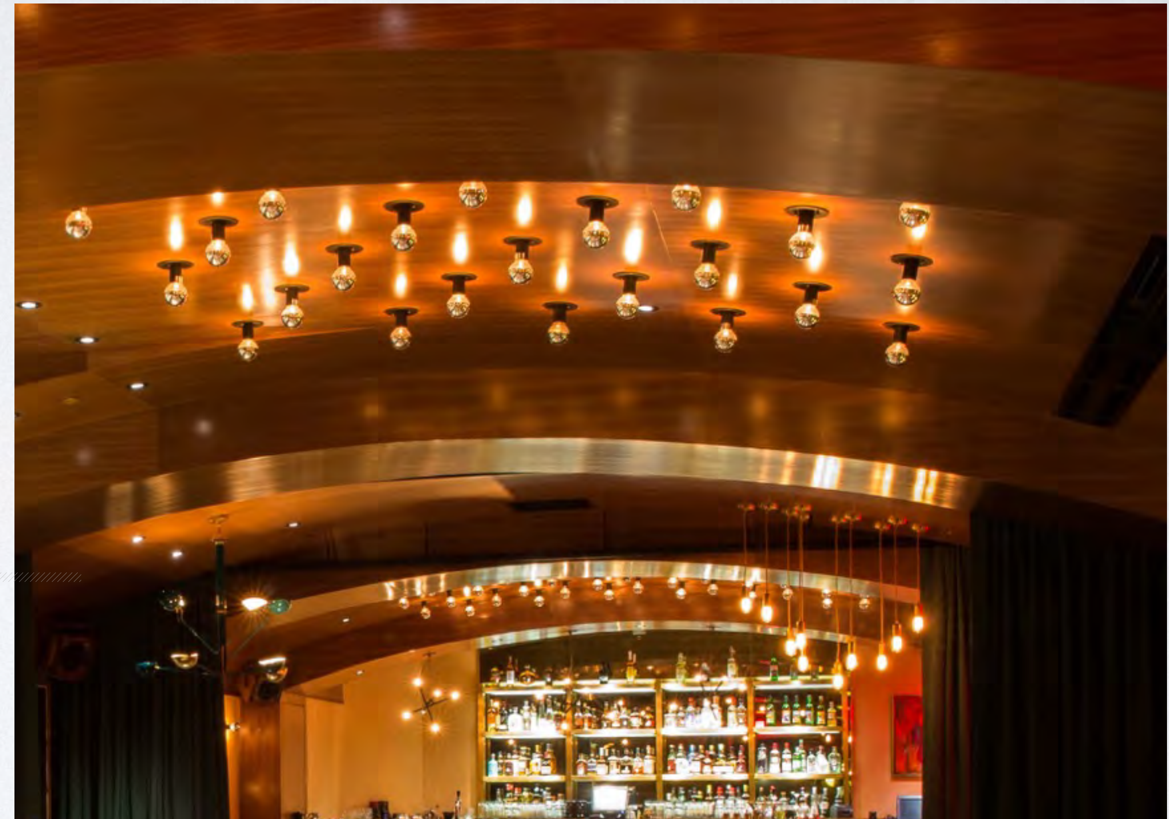
SINGLE DOME ARC - LEADING TO MAIN BAR ROOM - WOOD SUBSTRATE
